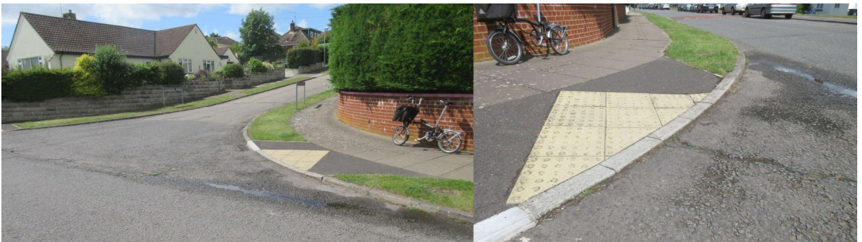
Footway crossing entrance from Bishopdown Road from Anderson Road. The road surface is poor, and the drop kerb is not flush with the road surface.
