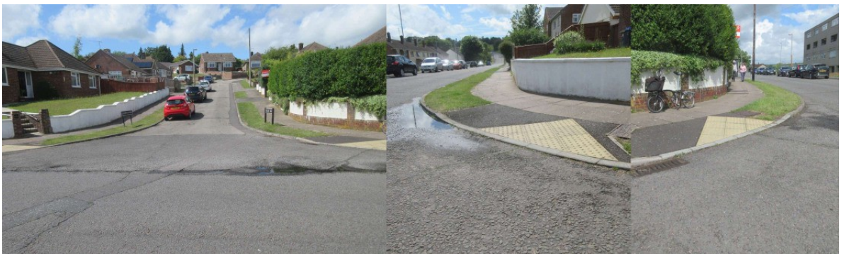
Entry of Bingham Road from Bishopdown Road. Poor road surface and drop kerbs not flush with road surface.
